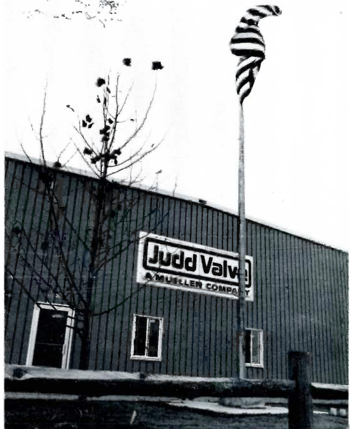
Judd Valve is the first Mueller company to display the new company logo on its sign. The new look for Mueller plants and subsidiaries' signs will soon be in evidence in all Mueller locations.
